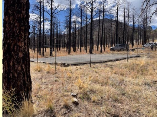
Completed trick tank
