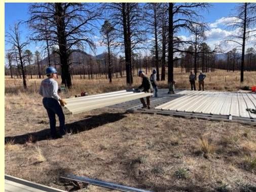
Apron under construction
